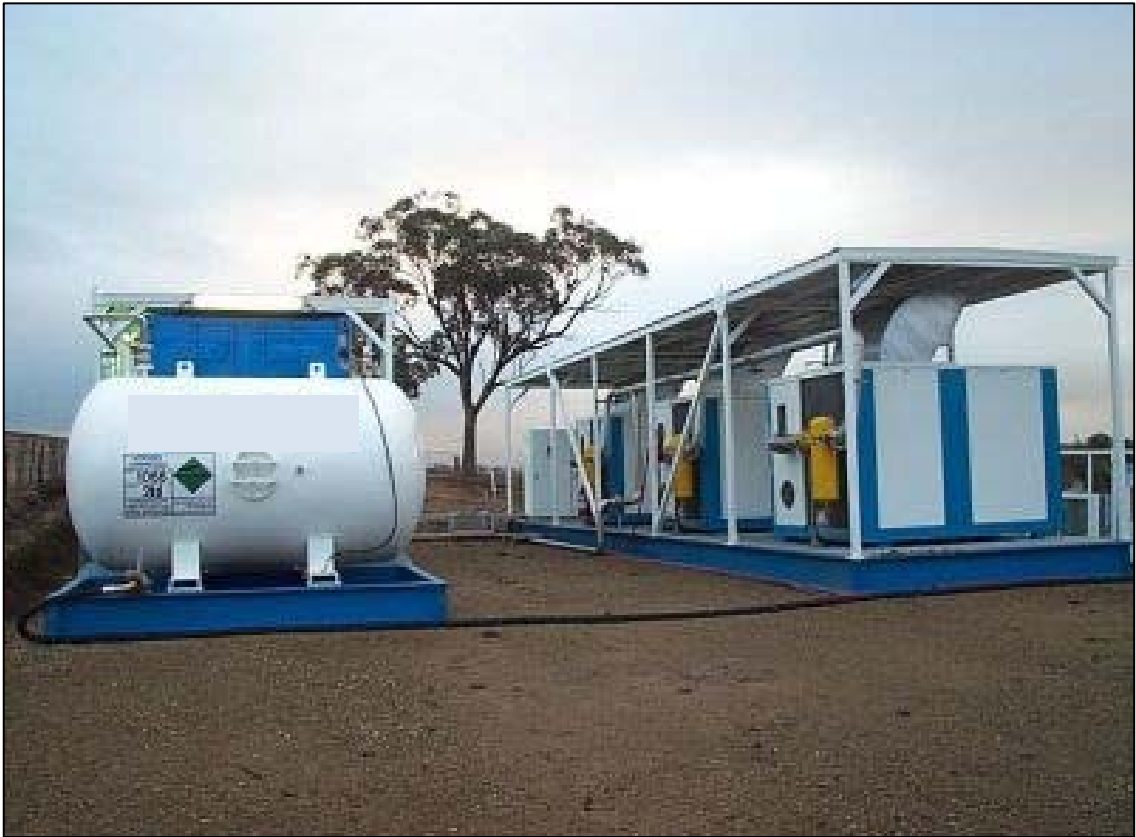
Figure 31: Membrane Separation Generator technology
