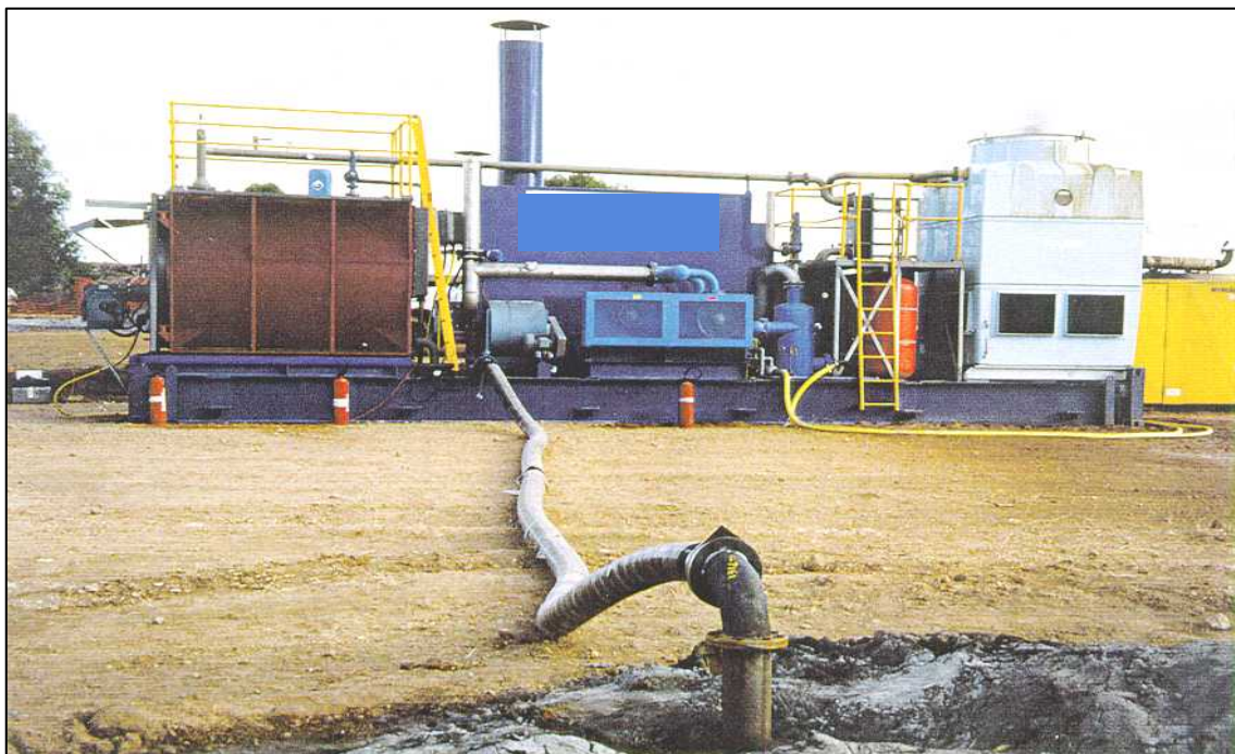
Figure 32: Tomlinson Boiler unit discharging down a borehole
