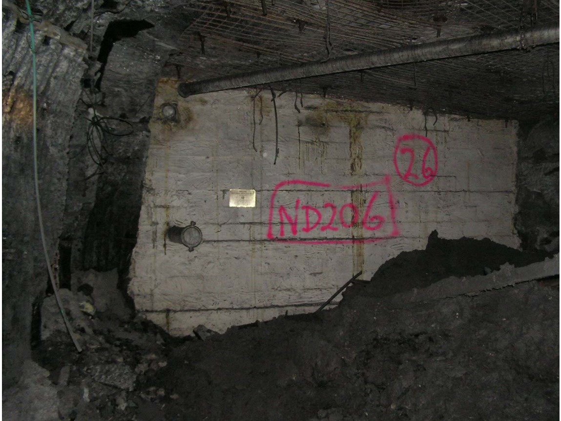
Figure 11: Stowage against goaf stopping impeding access
